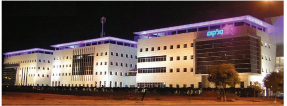
Cellcom Telecommunications, Inc. • Netanya, Israel
